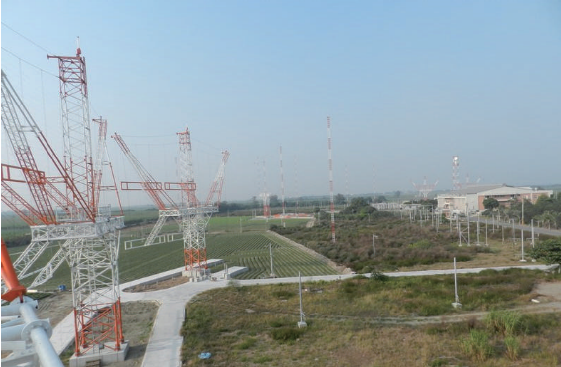
■ 央廣褒忠分臺建置短波高增益幕形天線 Curtain antenna at RTI Paochung branch
